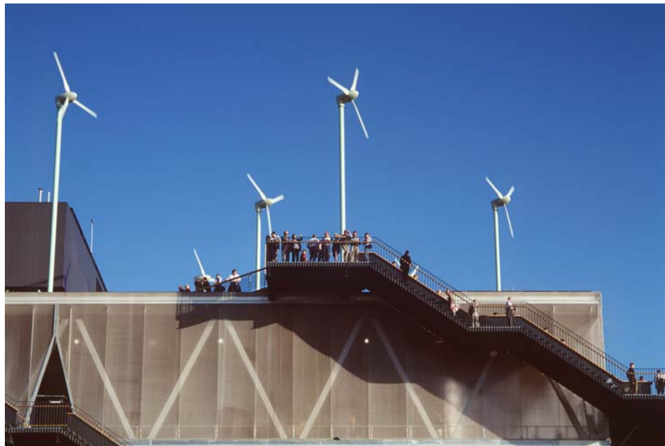
Tulipo's on roof of 6 storey Dutch Pavilion, Expo 2000, Hannover, Germany.
