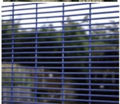
TRI-TEX or 'prison fence' as it is commonly known is a security mesh fencing system with narrow apertures. This prevents the 'would be intruder' having any foot or finger holds therefore making it extremely difficult to climb. TRI-TEX panels are overlapped at each post and secured by a full length clamp strip, domed headed bolts and permacone security fixings. The introduction of colour has now made the TRI-TEX mesh system a popular choice when security is paramount.
